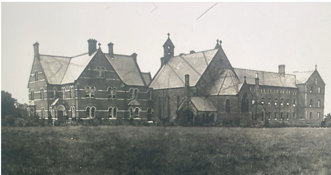
Convent of the Good Shepherd Marianville, Ormeau Road, Belfast (1990), photo T.2418/1/231, used with permission of the Deputy Keeper, Public Record Office of Northern Ireland (All that remains of the laundry is the chimney, which is now to the rear of apartments constructed on that part of the site.)
